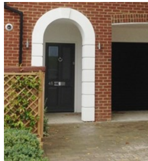
Recessed door and stuccoed arch give this entrance dignity and presence.
